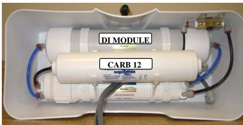
2. Remove the retaining clips from each end of the Aquathin Carb 12 pre-filter, then remove the tubing itself. You will feel some resistance as the tubing slides away from the O-ring inside the fitting.
